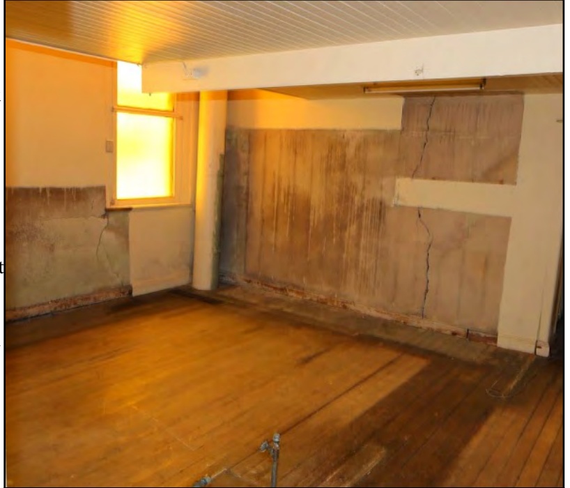
The gutted sacristy and covered nave entrance signify a season of renewal for St. Peter's that goes beyond our physical plant.
