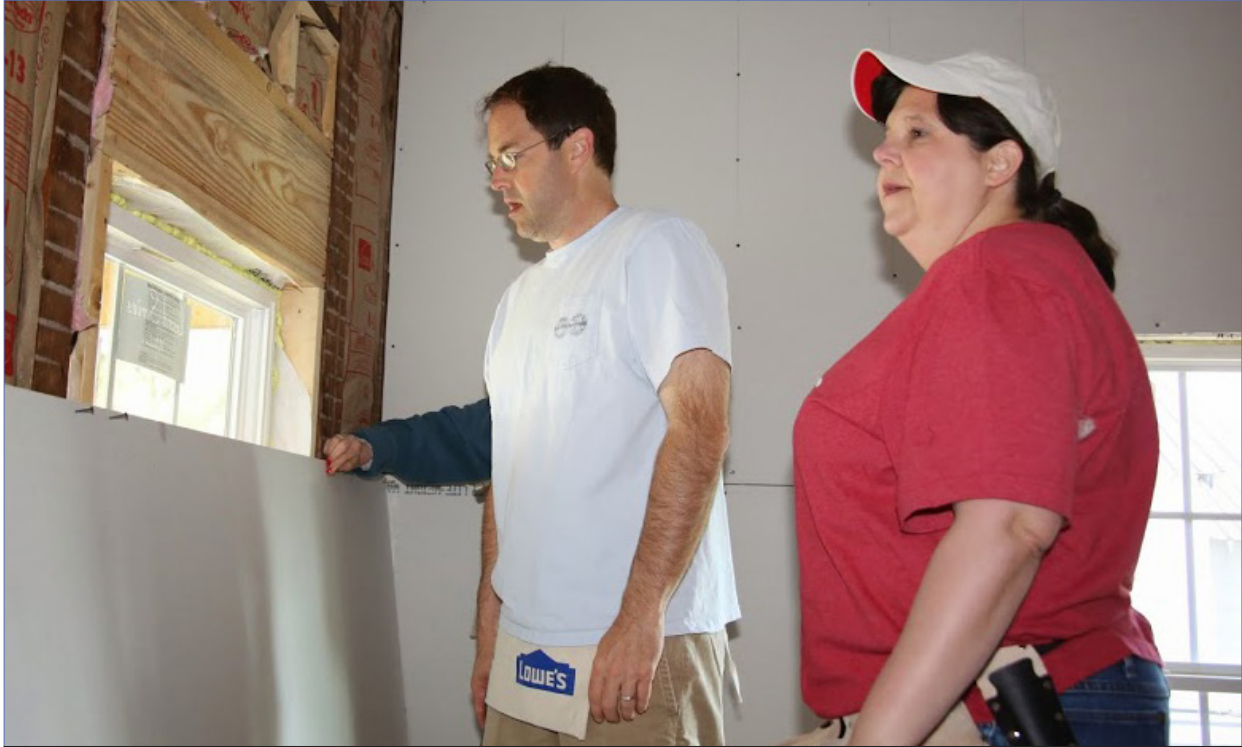
Andy Anderson & Leigh Patterson prepare to hang a piece of sheet rock during the build.
